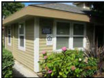
Bee Street Housing at 408 Bee Street in Sausalito. 6 units professionally managed by EAH.
