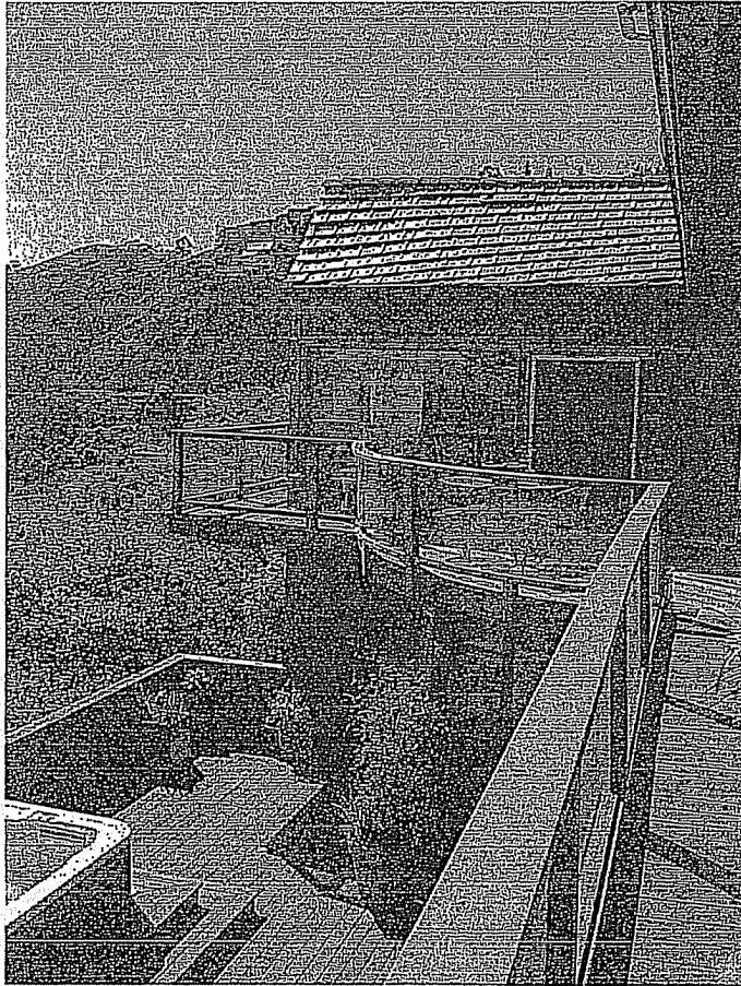
Back of House (from deck)
