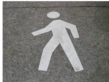
Bicycle and pedestrian pavement markings show where users should be on the pathway
