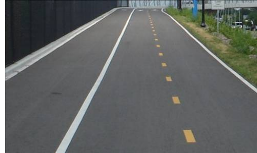
Recommended path striping shows a yellow skipped stripe dividing bicycle travel lanes and a white solid stripe demarcating the pedestrian walkway
