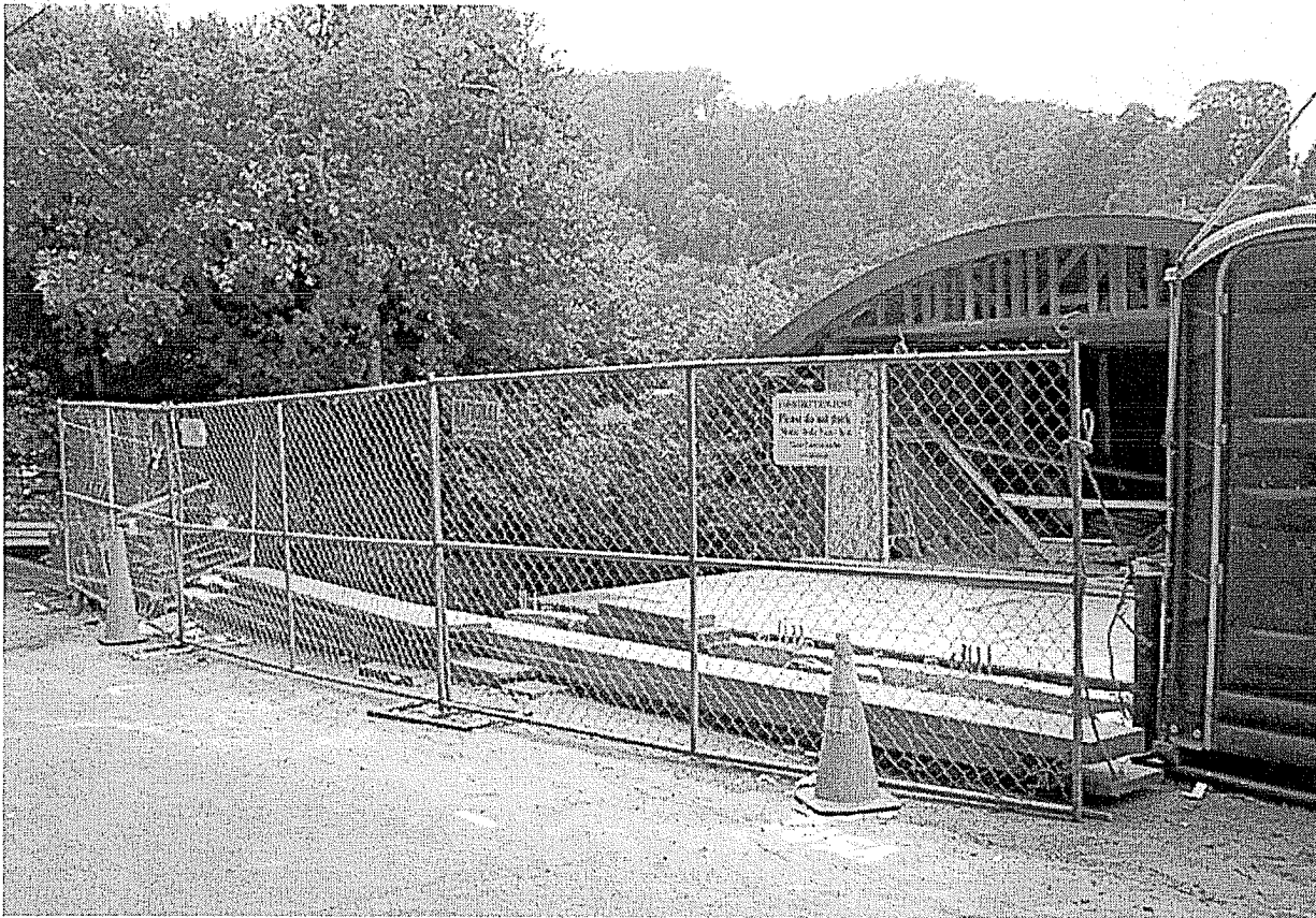
View of project during construction (November, 2007)
