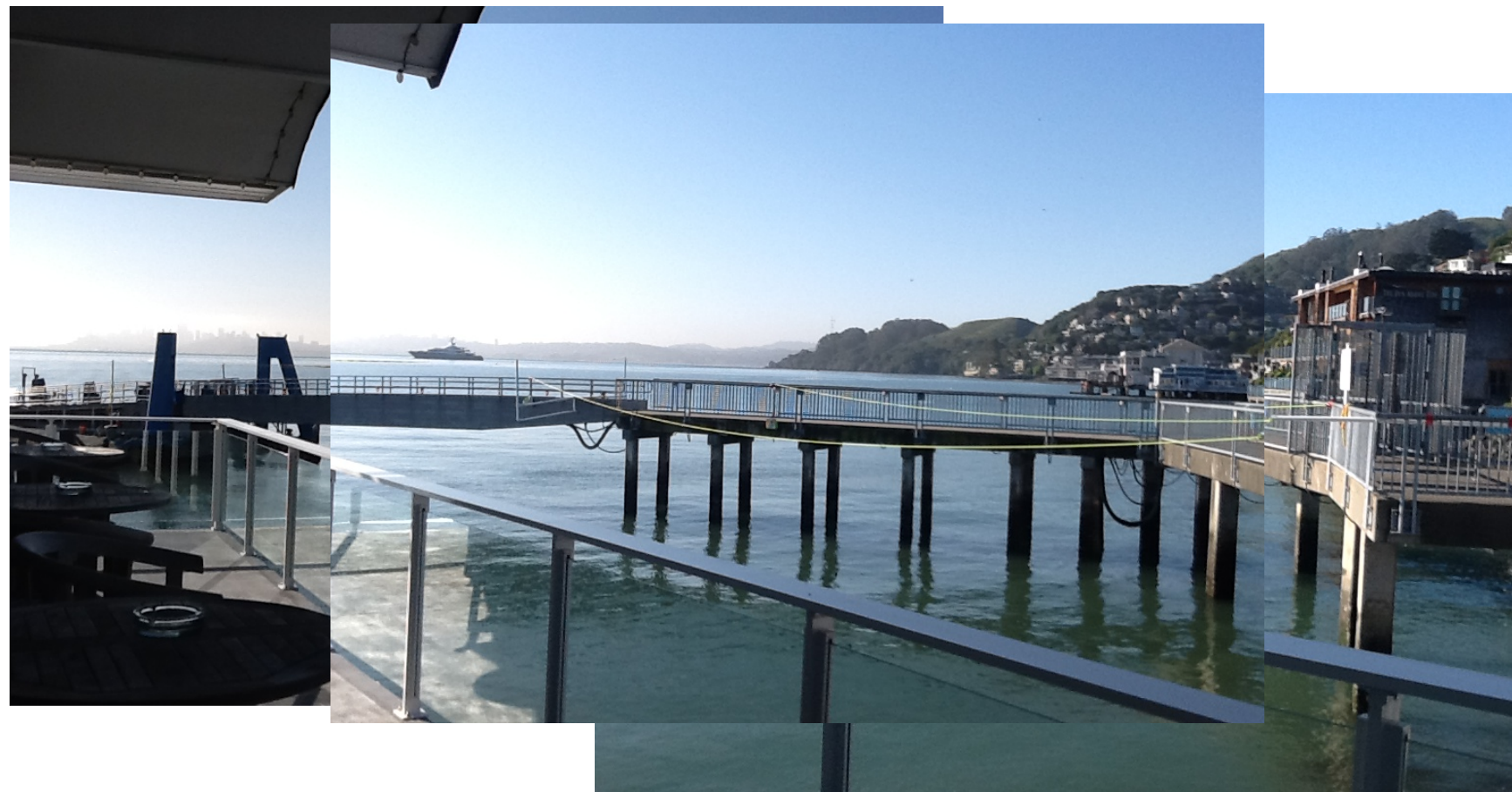
Staff photographs of view from southwestern corner of Sausalito Yacht Club (SYC) deck with story poles showing new access pier and gangway
