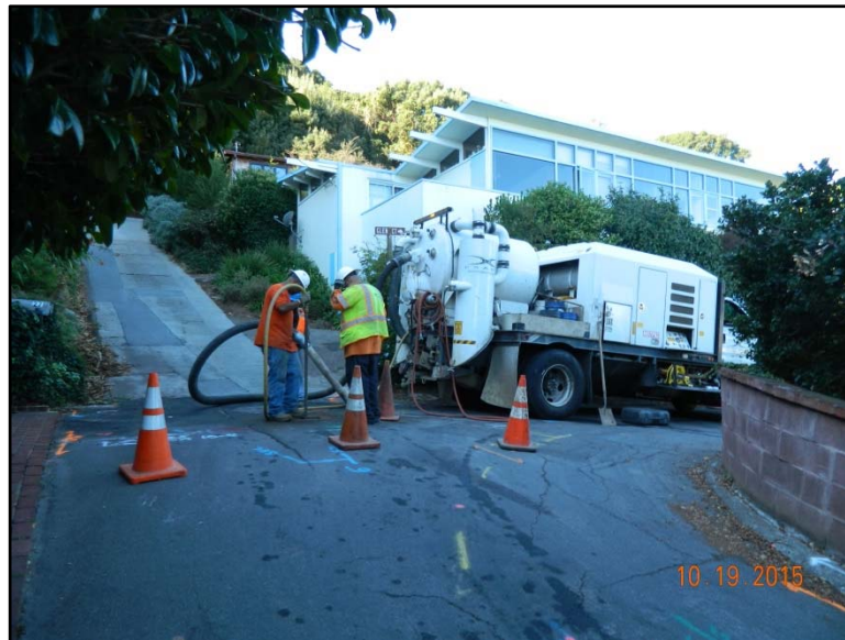
Photo 3 - Exaro crew at pothole location No. 2.
