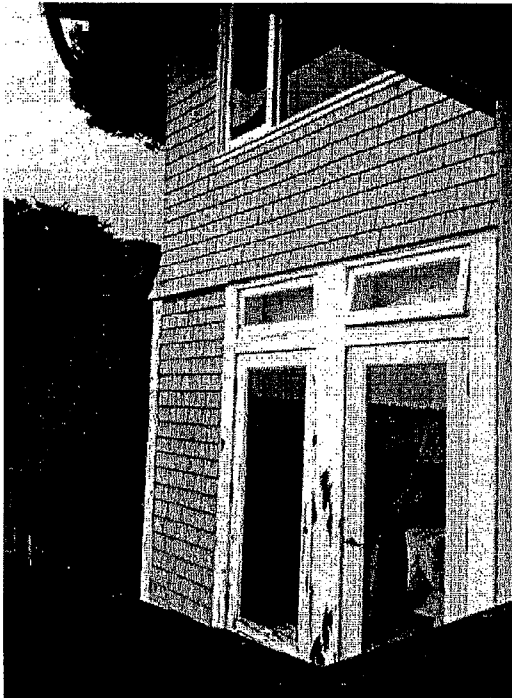
Exhibit F: Southeast Corner
