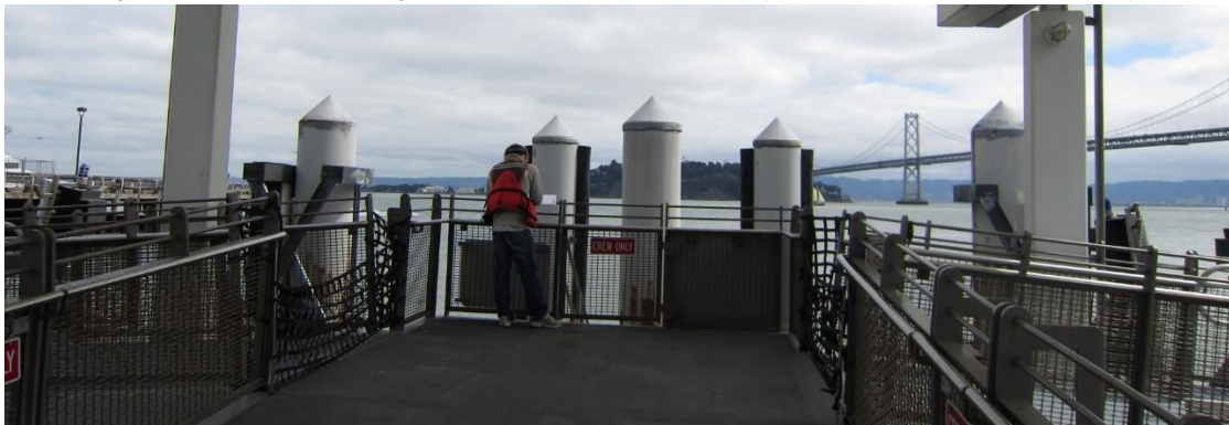
Figure 3 – San Francisco Downtown Ferry Terminal Gate E – Fabric Mesh Gate
