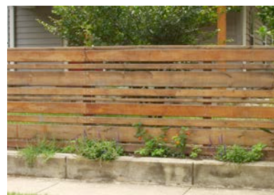
CLEAR WESTERN RED CEDAR W/ CLEAR STAIN - SEALER WOOD SLAT PRIVACY FENCE
