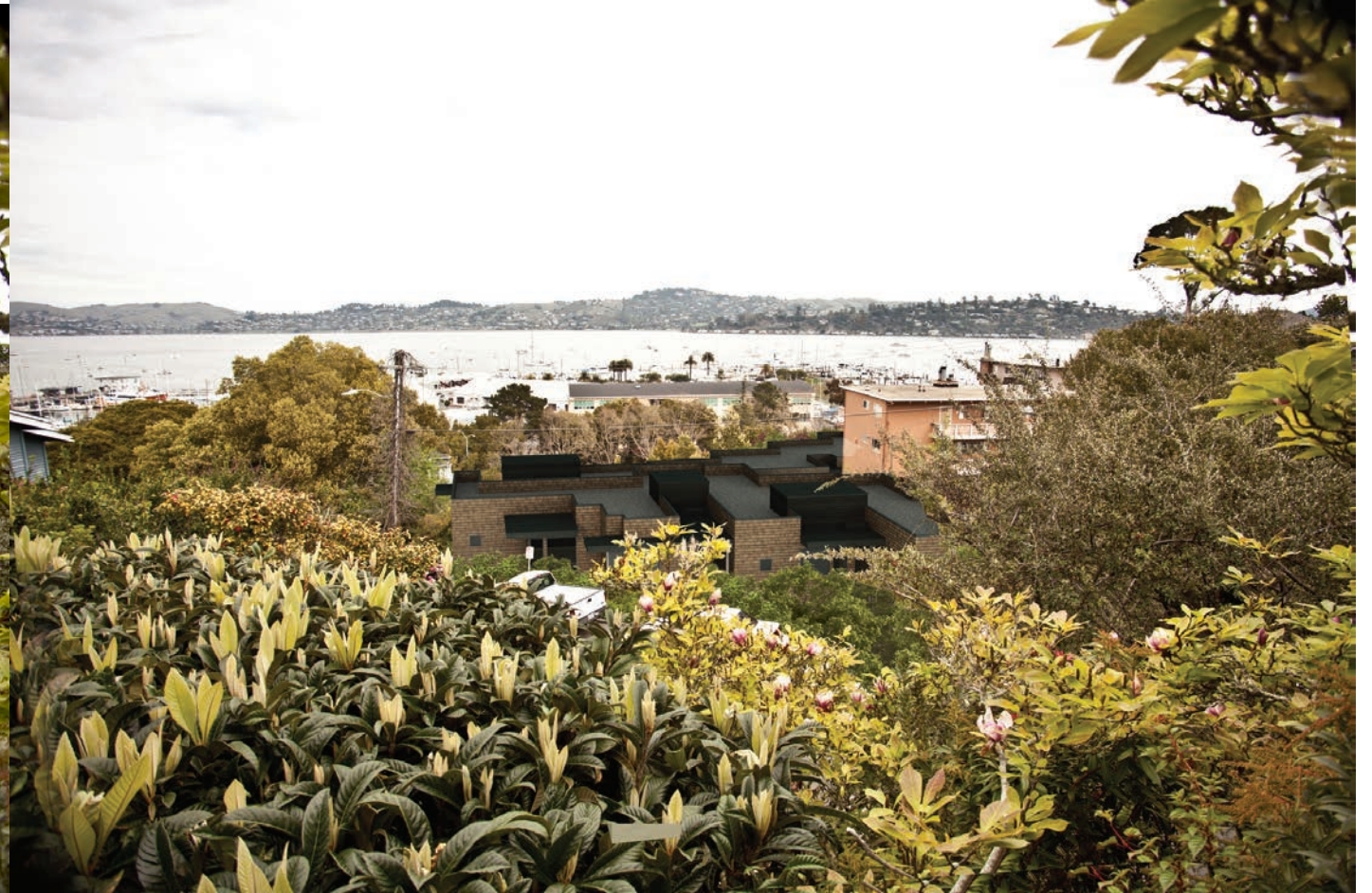
VIEW OVER PROJECT AFTER CONSTRUCTION
