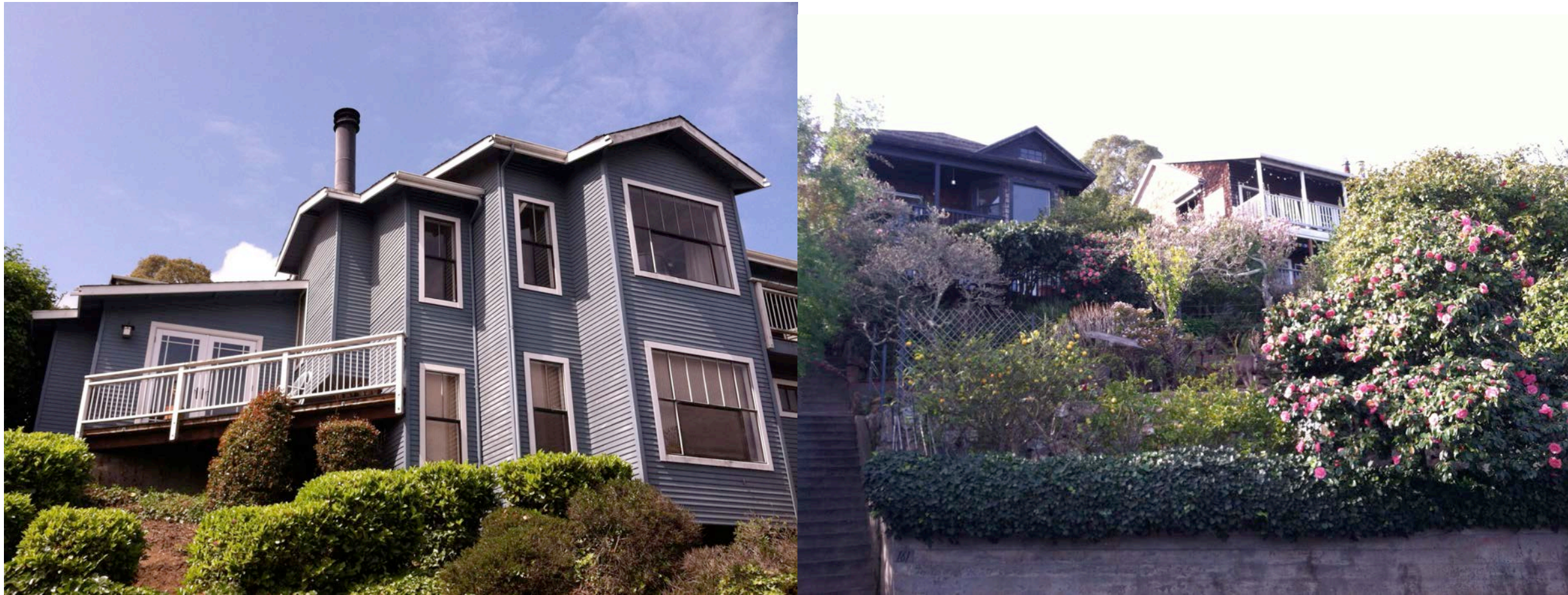
HOUSES ABOVE SITE ON FILBERT
