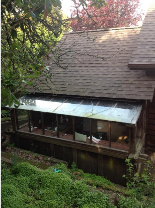
Figure 16. Glass and wood frame portion of façade.
