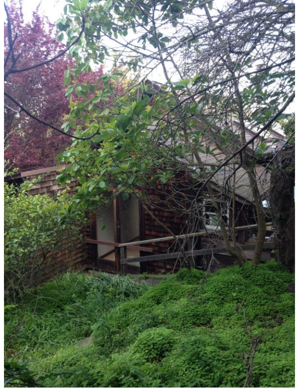
Figure 12. Rear façade, looking northwest.
