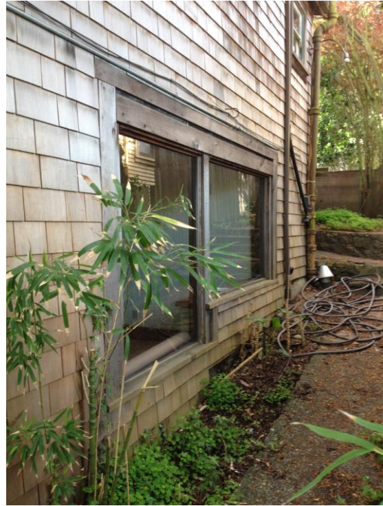
Figure 7. Irregularly paired windows.
