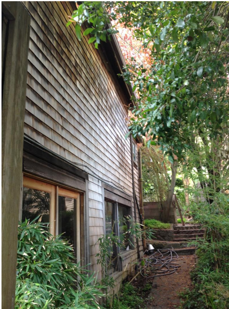
Figure 5. Northwest façade, looking south. Recessed addition is not visible.
