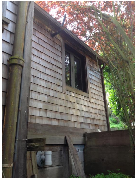
Figure 9. Rear addition, foundation and first story level.
