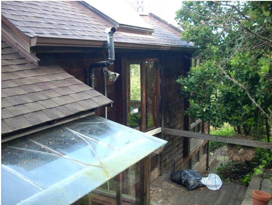
Figure 15. Southeast façade, looking north.
