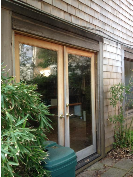
Figure 6. Basement level doors.
