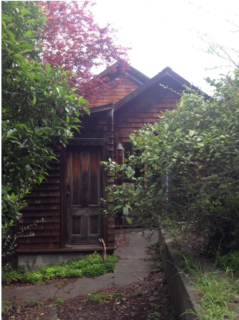
Figure 10. Rear façade, looking northeast.
