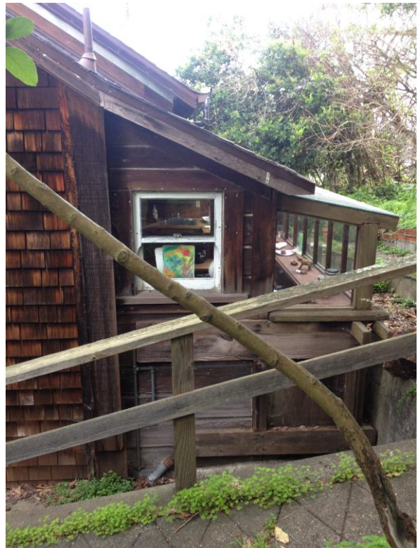
Figure 14. Right (south) side of rear façade.
