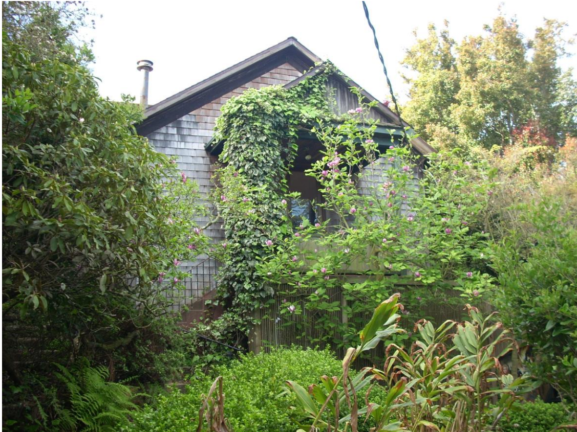
Figure 2. Primary façade of 1745 Bridgeway, looking southwest.
