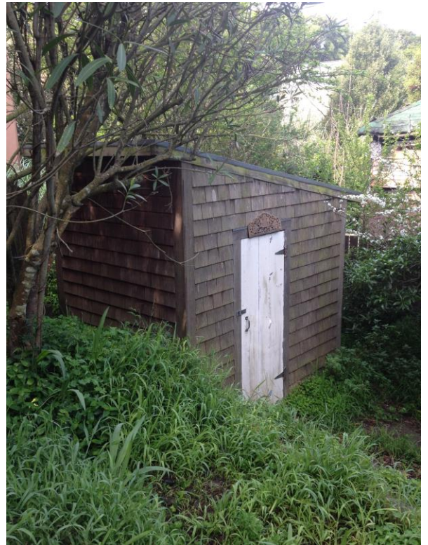
Figure 21. Shed at rear property line.
