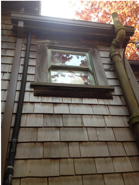
Figure 8. First story double hung window and lowered roof section.
