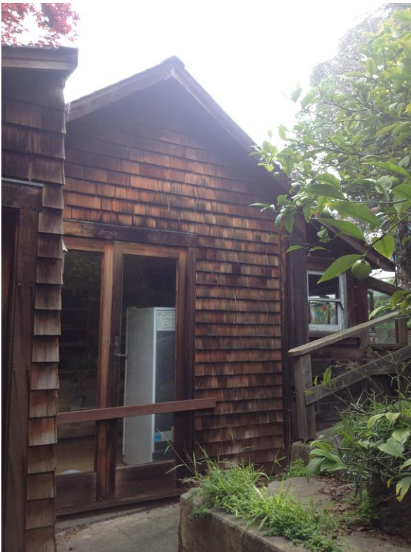
Figure 13. Center portion of rear façade.
