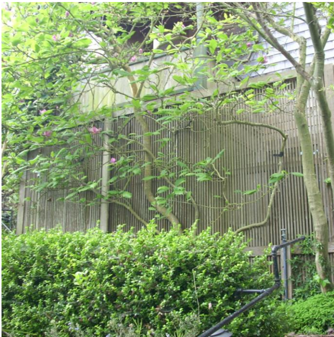
Figure 3. Wood slat screen at basement level of primary façade, looking south.
