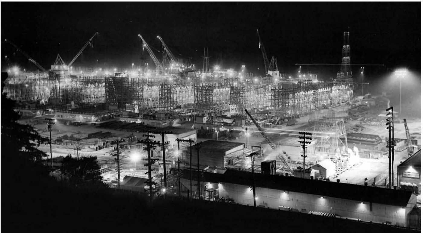
Marinship construction at night, circa 1942
