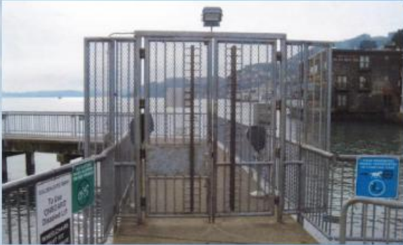
Existing Gate Steel Swing Gate with Diamond Pattern Grating
