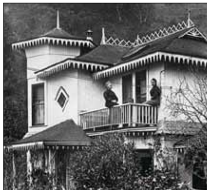
Eclectic Carpenter Gothic details are visible on both of these buildings.
