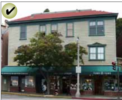
Upper photo: Original condition; note single, double-hung windows at right edge of facade.
