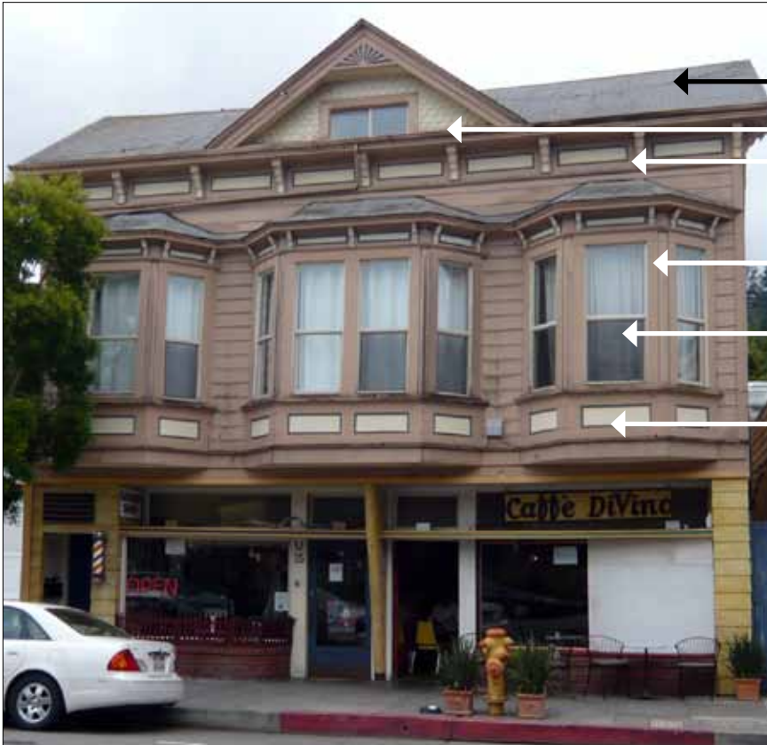
This storefront is a hallmark of mixed styles. This building combines Italianate and Queen Anne features. The upper floor retains many of this buildings character-defining features, whereas the lower floor storefront has been modified.
