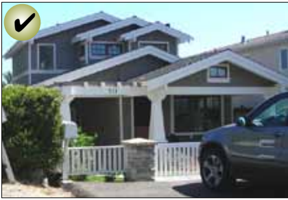
Position taller portions of a structure away from neighboring buildings of lower scale.
