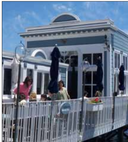
Italianate commercial style details include elaborate cornices, with decorative brackets and banding.
