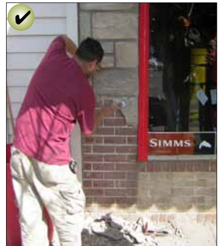
Consider removing later covering materials that have not achieved historic significance. Once the non-historic siding is removed, repair the original, underlying material.
