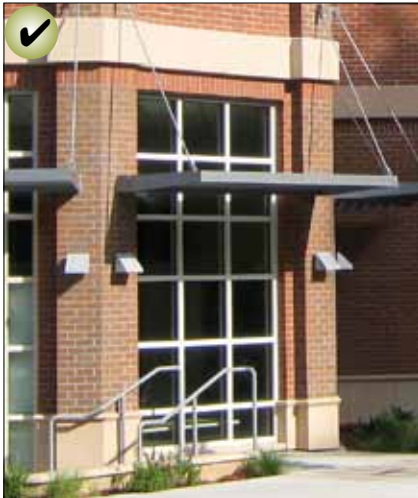
Use exterior or facade integrated (seasonal) shading devices to block direct summer sun.
