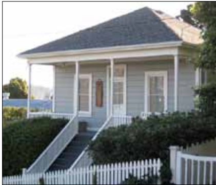
The influence of the Bungalow style is visible on these buildings. Key features include double-hung windows, wood siding, hipped shaped roof and porch.
