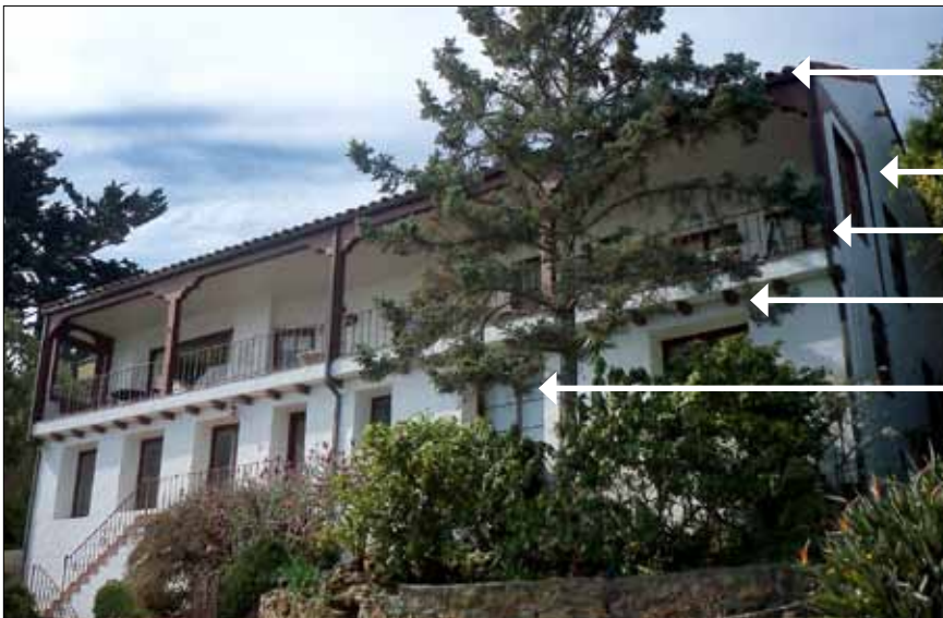
The influence of the Mediterranean Revival style is visible on this residence.
