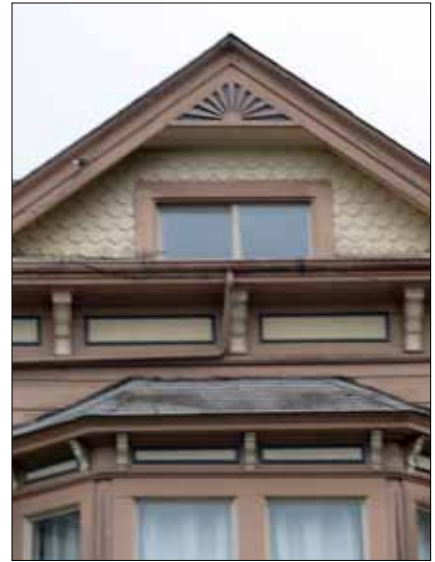
Sunburst jigsaw detail in gable end is a distinctive characteristic of the Queen Anne Style.
