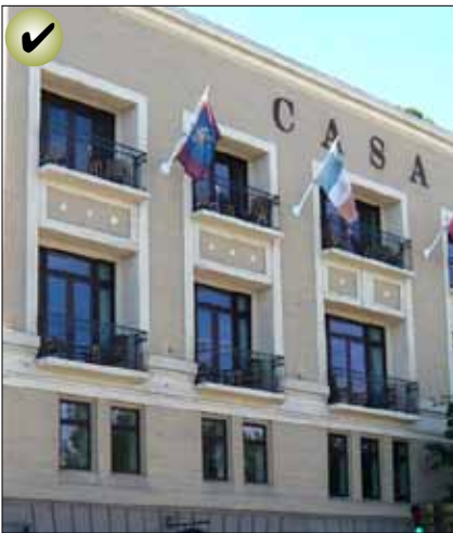
A balcony should be in character with the building and simple in design. Light wood and simple metal work are most appropriate.
