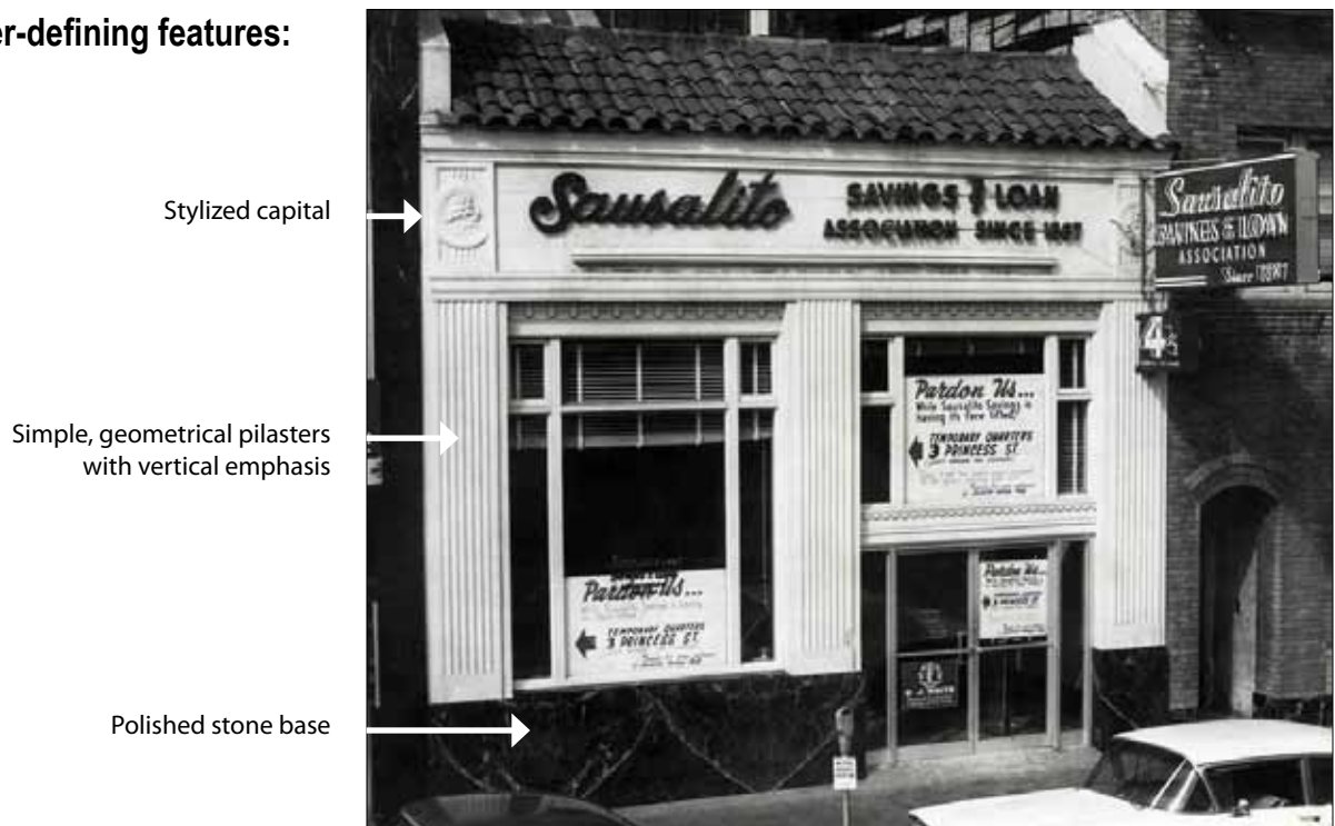
This building combines details of Art Deco with some Neoclassical motifs.
