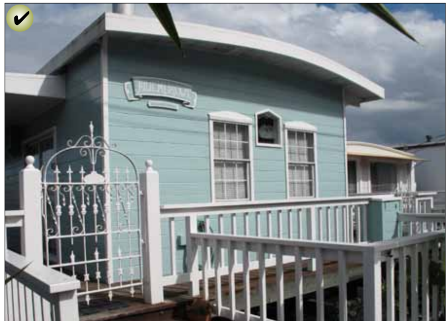
Preserve character-defining wood and metal materials. This includes the deck, railing, fence, siding and window trim on this Ark style waterfront building.
