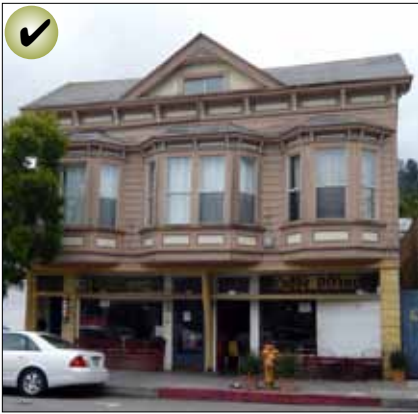
Preserve the original roof form of a historic structure.
