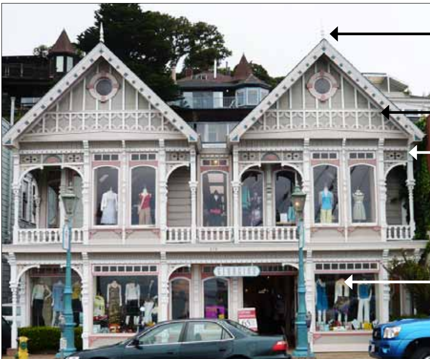
These cottages, originally part of a set of three matching Queen Anne designs, have been adapted to commercial uses, and some original features are therefore altered, but the ornamental bracket supports, strapwork detailing and variety of materials continue to reflect the original character.
