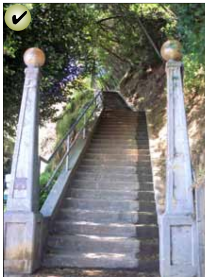
Preserve significant masonry and concrete features. Materials that were not painted historically should not be painted.
