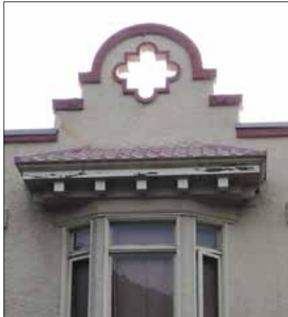
Stepped parapet with tile accents
