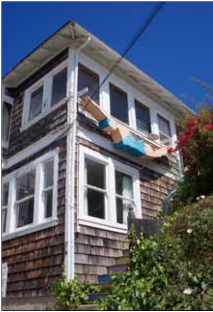
This building has several features that are characteristic of the Craftsman style. Key features include grouped double-hung windows, wood shingles and exposed roof rafters.
