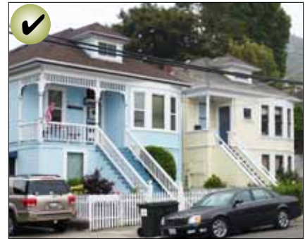
Maintain the existing location, shape, details and posts of an original porch.
