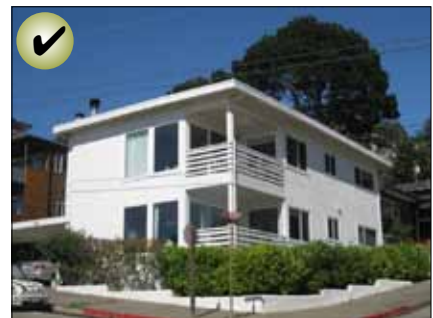
A porch is one of the most important character-defining elements of a facade. Preserve a porch in its original condition and form.
