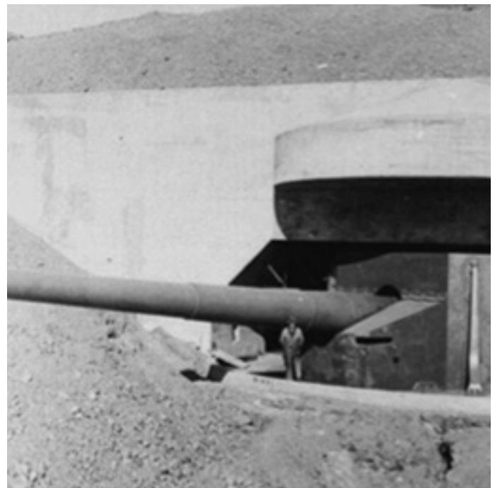
Battery Townsley, Fort Cronkhite, just after construction, c.1939
