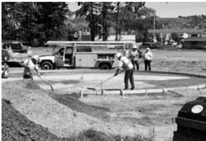
Workers installing foundation for Age Friendly Fitness Zone in MLK Park
