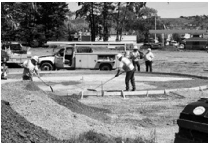
Workers installing foundation for Age Friendly Fitness Zone in MLK Park
