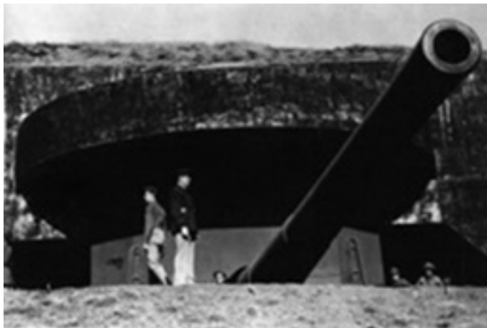
Soldiers stationed at Battery Townsley located at Fort Cronkhite in the Marin Headlands. The battery was completed in 1940. Photo: PARC, Golden Gate National Recreation Area
