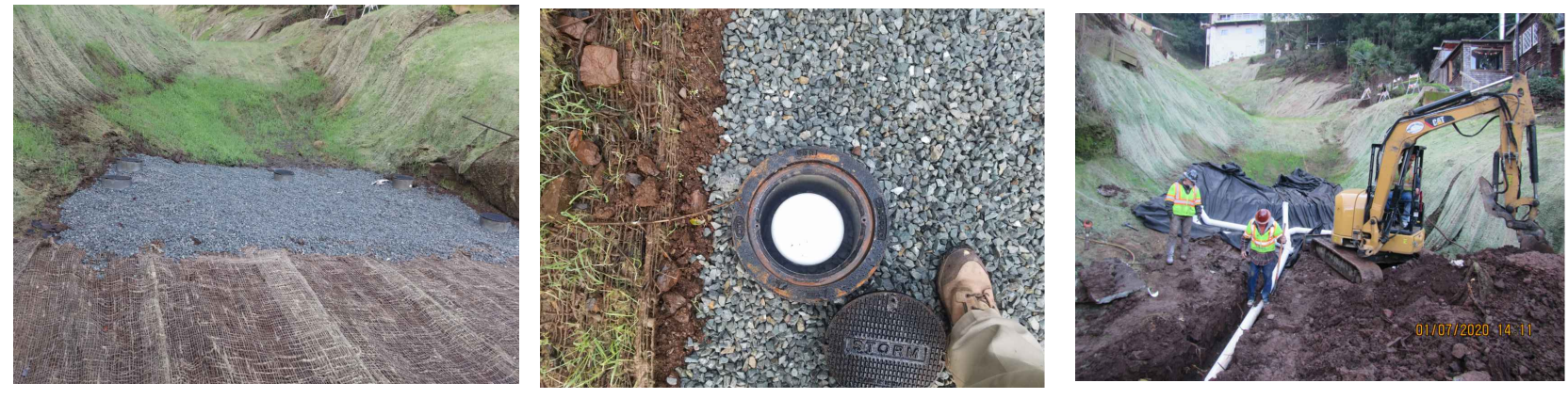
PHOTO #3 PHOTO #4 PHOTO #5 PERMEABLE GRAVEL BED/SDCO AND SUBDRAINS
