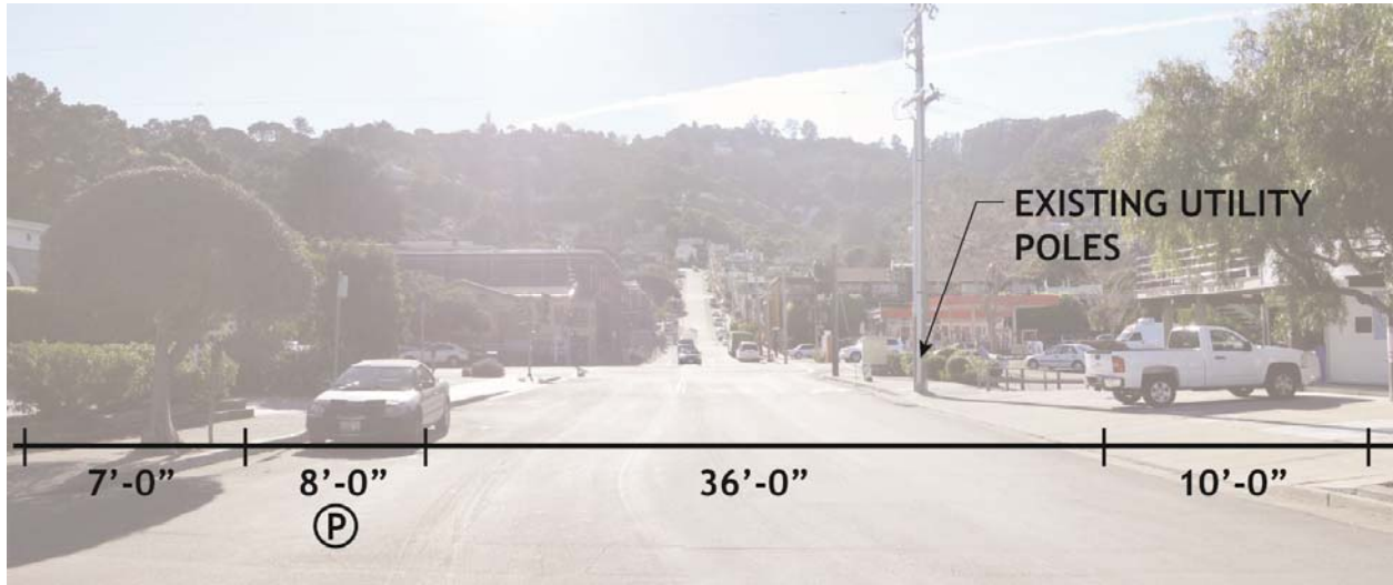
Figure 7-20 Segment 1G Johnson Street Existing Conditions
