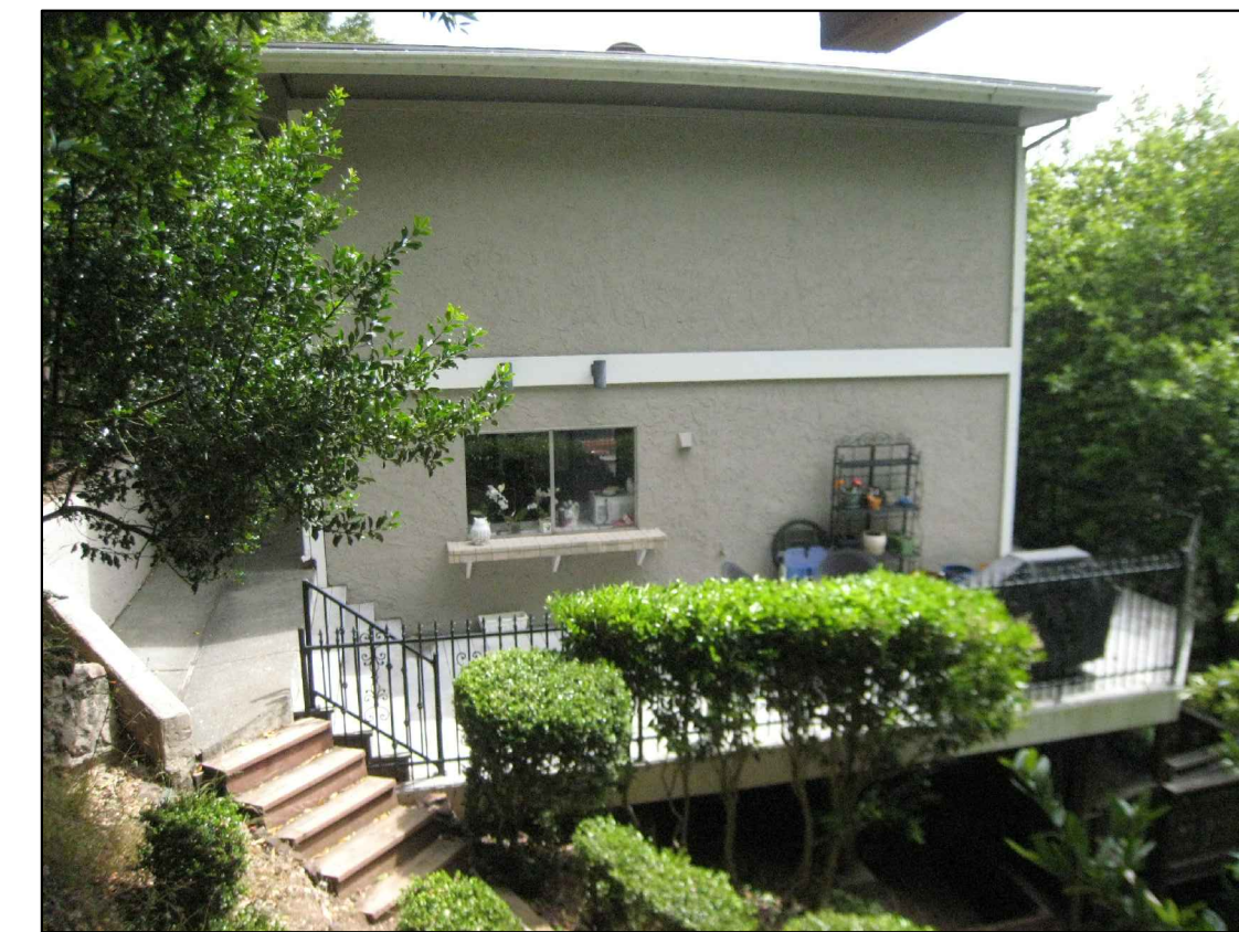
EXISTING REAR DECK AT MAIN HOUSE
