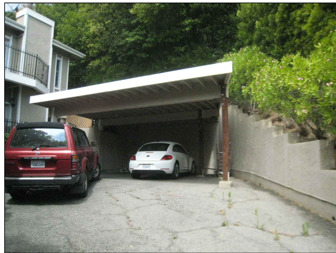
EXISTING GARAGE ROOF
