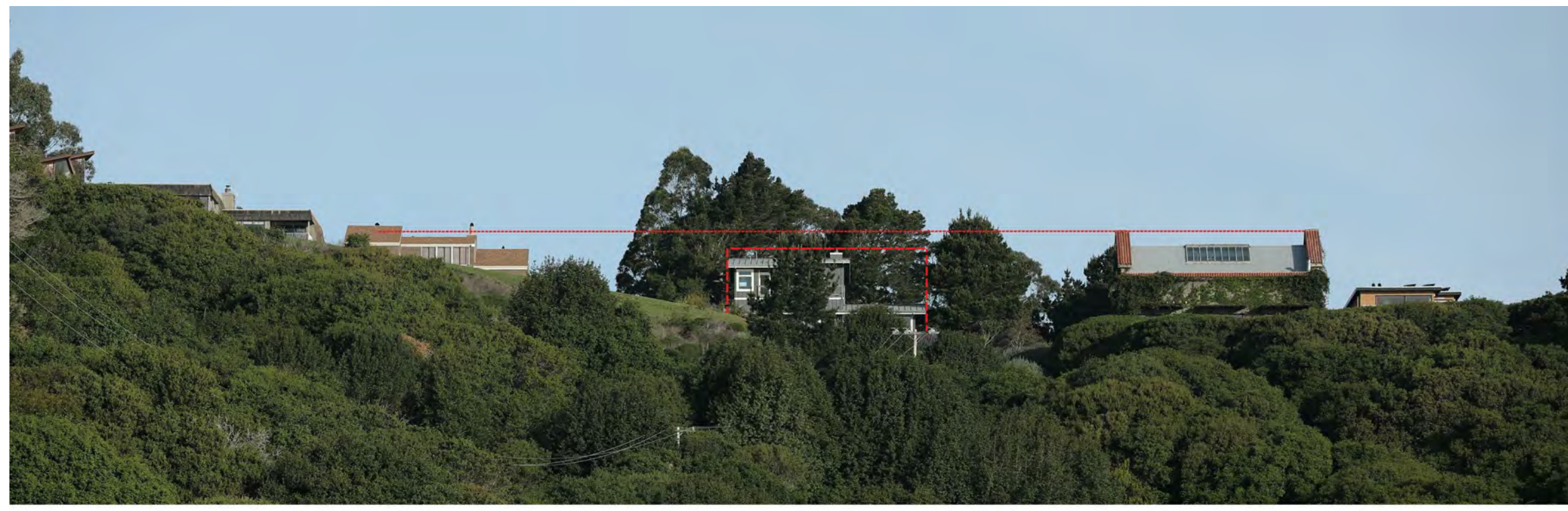
EXISTING / 3 MARION AVENUE, SAUSALITO / SOUTH FACADE FROM GGNRA
