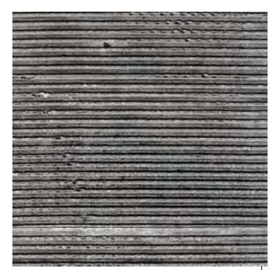
RIBBED CONCRETE SPECIFIED WHERE SLOPE IS >18% Per Fire Prevention Department, where slope is in excess of 18% shall be Ribbed Concrete
