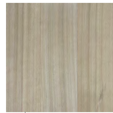
CLEAR CEDAR / THIRD FLOOR CEILING & ENTRY CANOPY
