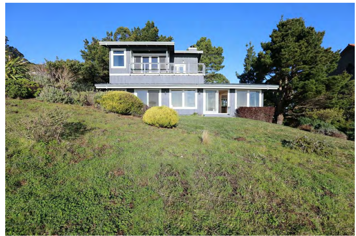
IMAGE 1 EXISTING / SOUTH ELEVATION FROM GGNRA
