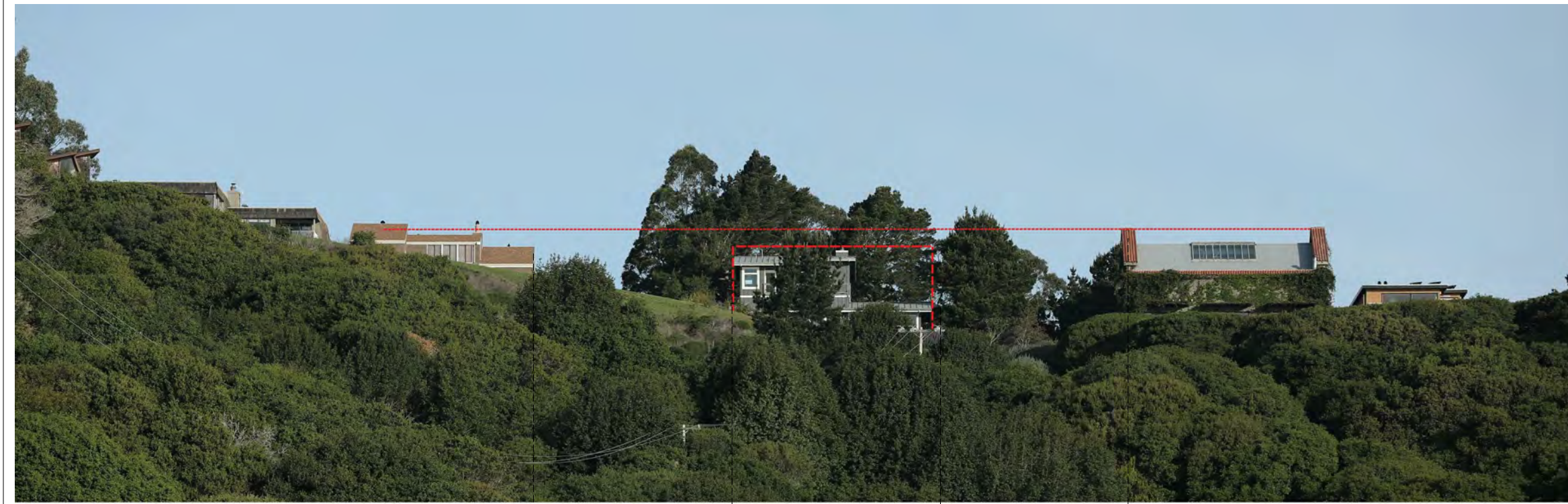
SOUTH FACADE FROM GGNRA / EXISTING
