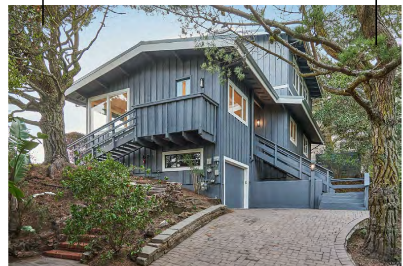
IMAGE 6 / VIEW LOOKING AT NORTH - EAST ELEVATION
