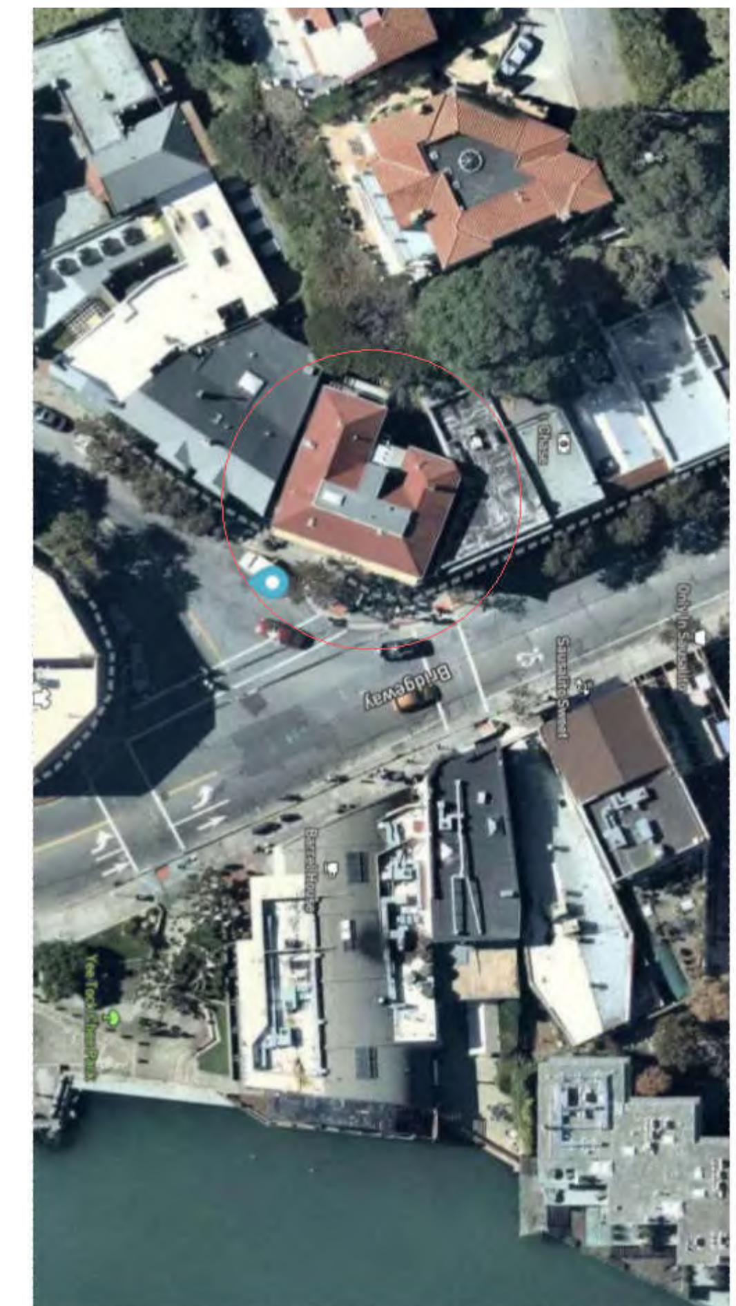
6 PRINCESS STREET AERIAL VIEW
