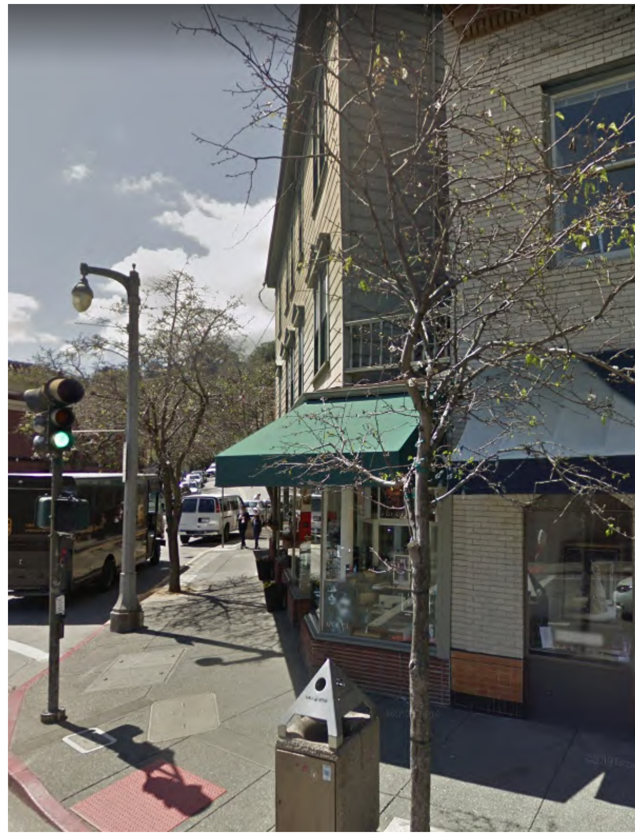
6 PRINCESS STREET SIDE VIEW 2017 (NOTE AWNINGS)
