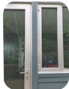
[E] HARDPLANK SIDING AND TRIM, AND ALUMINIUM WINDOWS AND DOOR AT SOUTH ELEVATION
