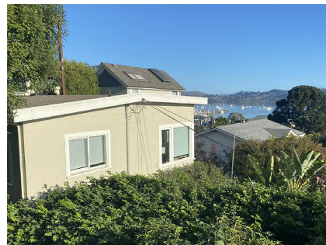
424A LOCUST EAST FACADE FROM 306 BONITA
