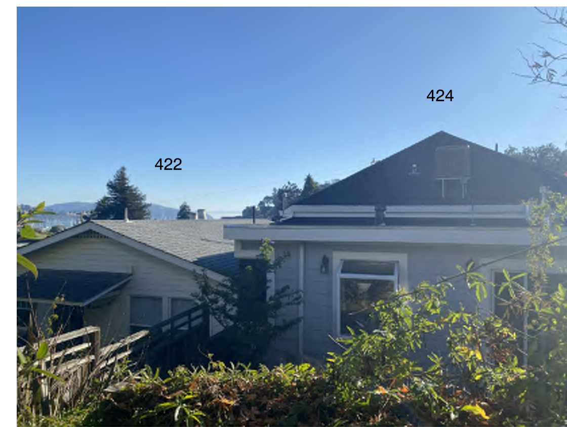
422 & 424 LOCUST FROM 424A LOCUST STREET
