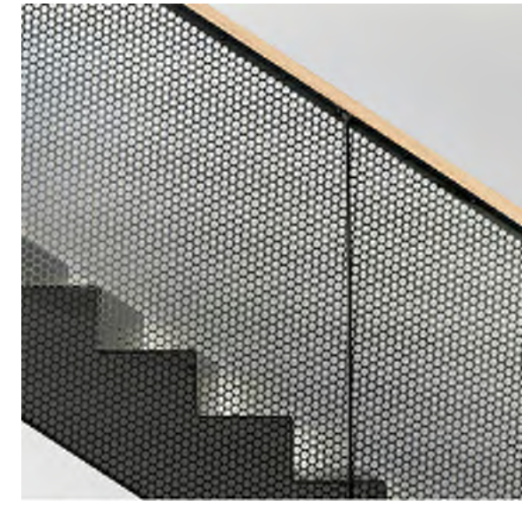
PROPOSED RAILINGS: STEEL & PERFORATED METAL PAINTED BLACK WITH WOOD CAP
