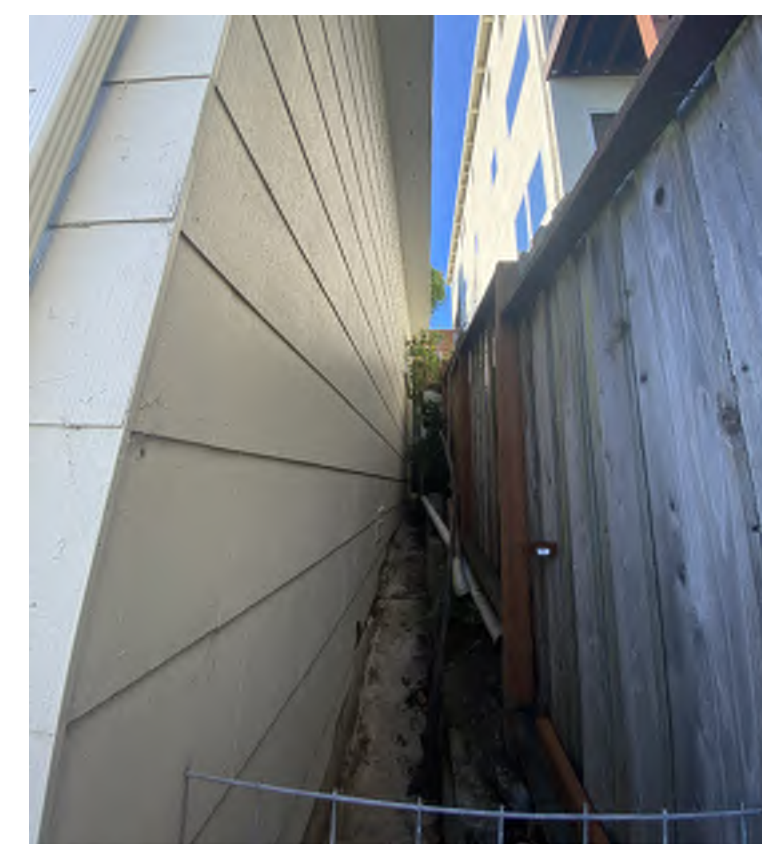
424A LOCUST - WEST FACADE
