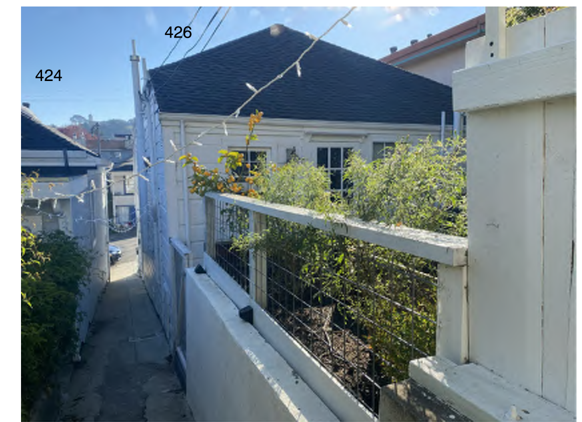
426 LOCUST FROM 424A LOCUST STREET
