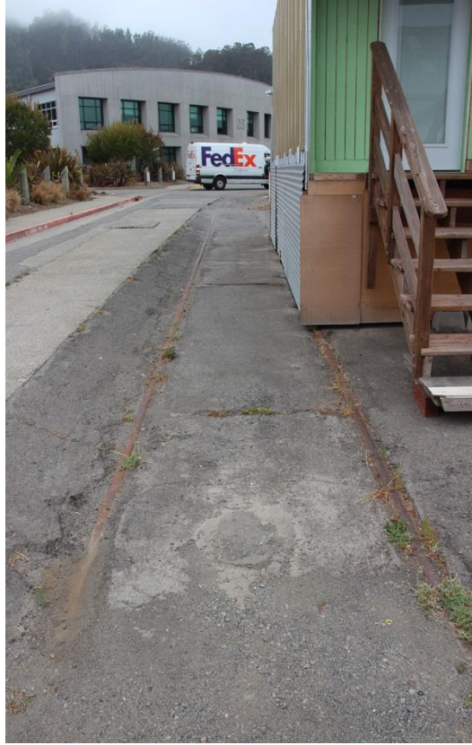
Figure 5. Track segment, looking southwest.
