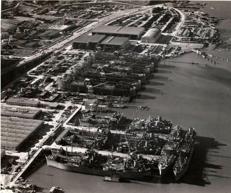
Figure 7. Marinship, 1944, looking northwest.
