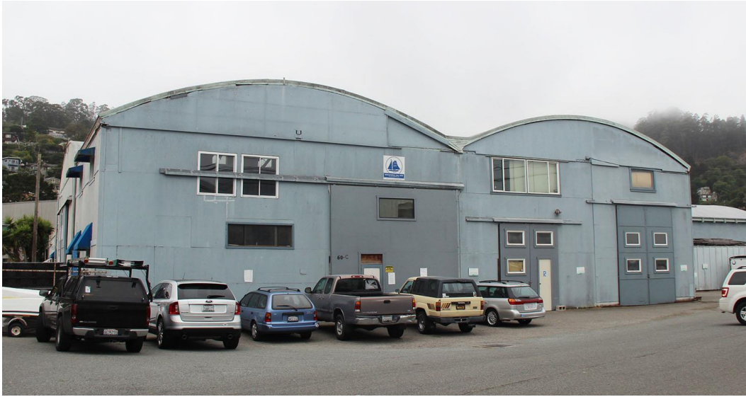
Figure 2. Building 13 at 60-70 Liberty Ship Way.
