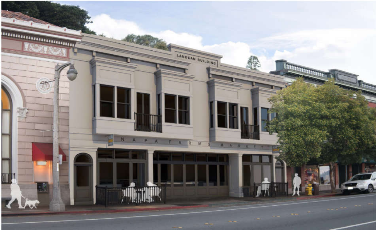
Figure 2: Rendering of Proposed Bridgeway Elevation (without Street Trees) Source: Michael Rex Architects
