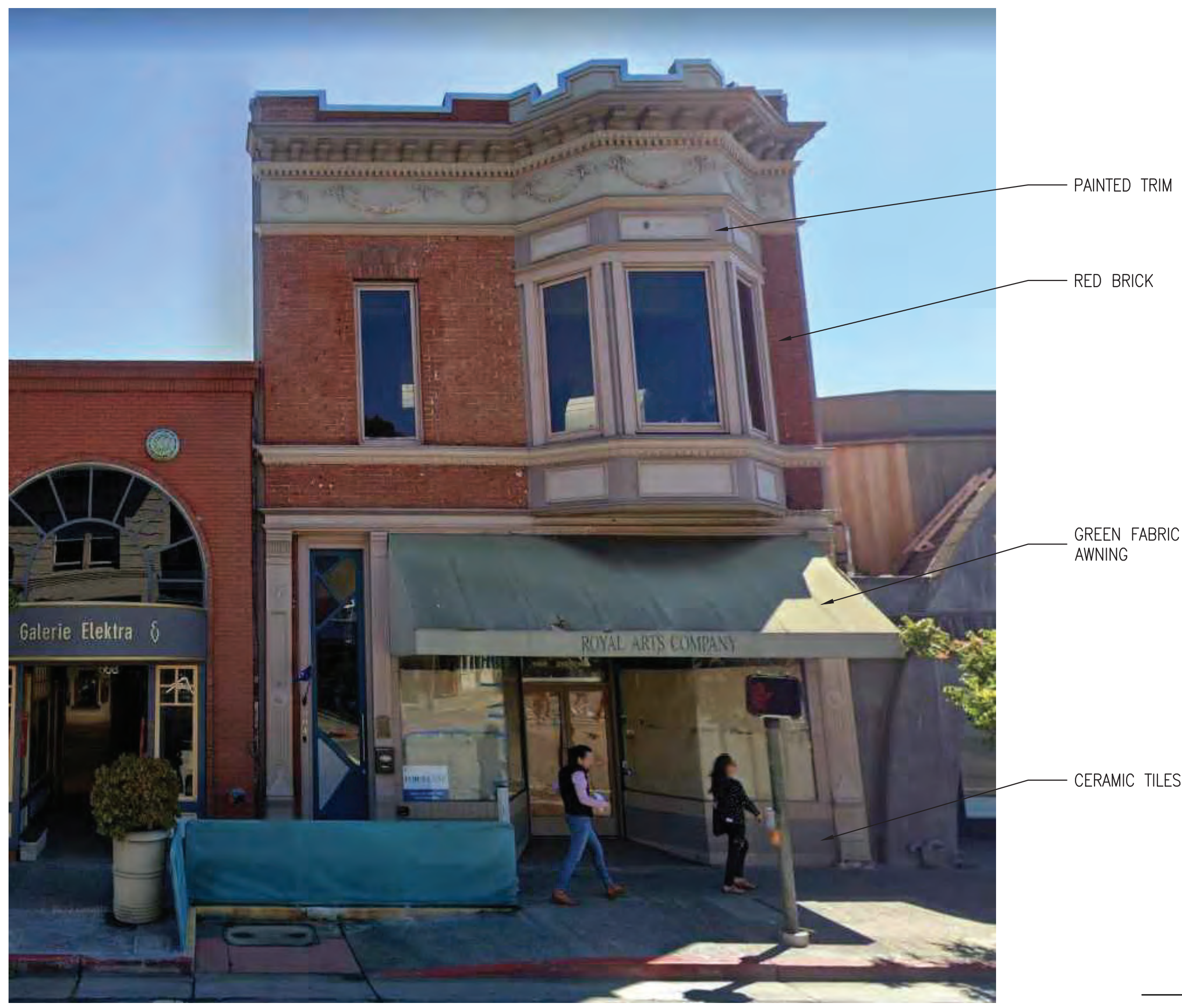
3 EXISTING STOREFRONT PHOTO WITH FINISHES N/A
