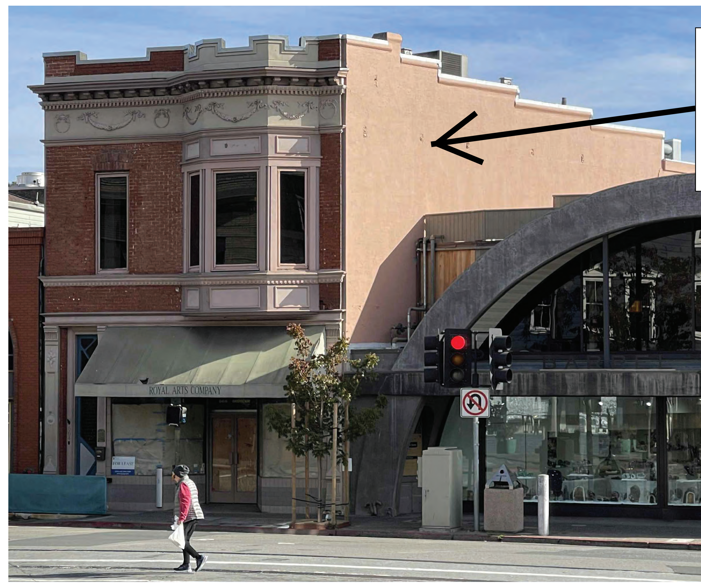
2 EXISTING STOREFRONT AND SIDE OF STORE PHOTO N/A
