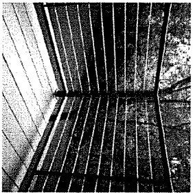
METAL I-BEAM STAIRCASE WITH STONE TREADS CABLE RAIL GUARDRAILS METAL POST & TOP RAIL
