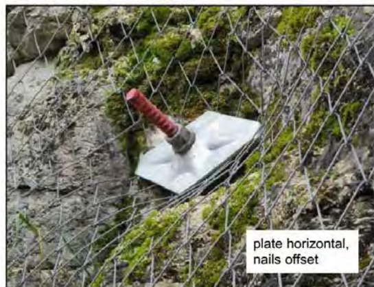
THE FINISHED TECCO® SYSTEM LAYED AND TENSIONED
