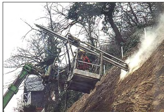
Example: Depending on terrain conditions, drilling work can also be carried out from a small crane platform or lifting platform.
