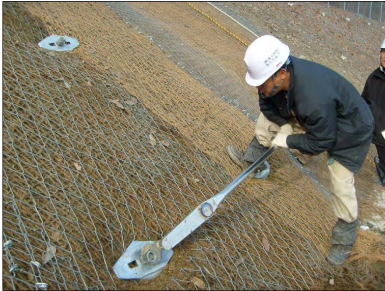
Tightening of the nut to the required torque using a torque wrench.
