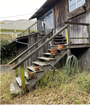
Stairs to be removed upper
