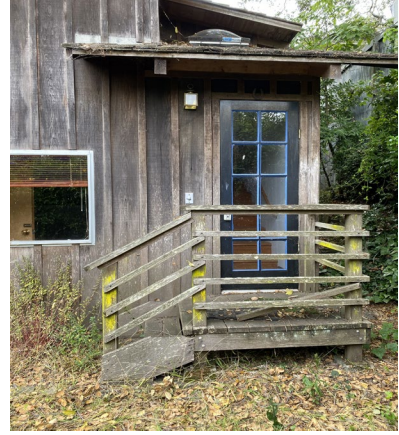
Stairs and deck to unit to be replaced
