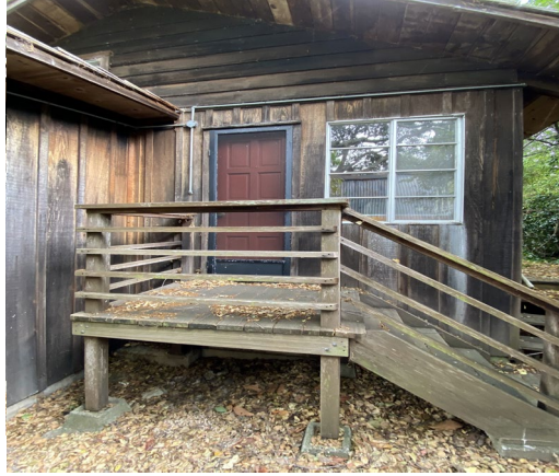
Stairs and deck in back right corner to be removed
