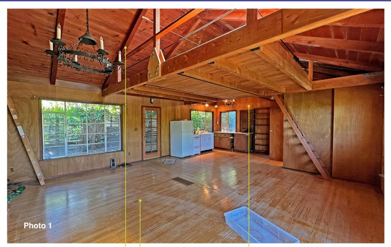
The second level ceiling is wood beams and wood planks.
