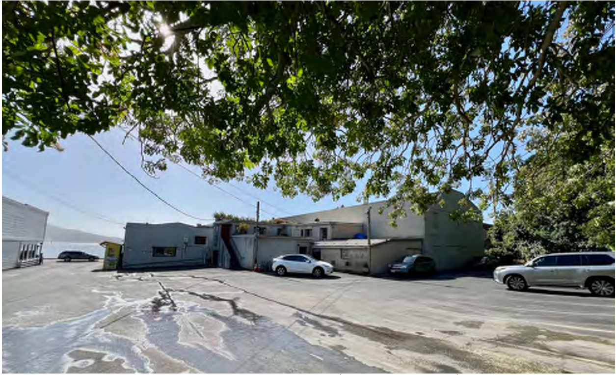
Figure 26: Subject parcel, looking east from parking lot (Turnbull May 2024)
