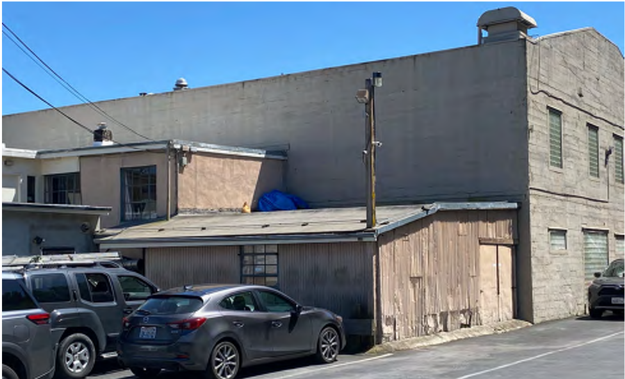
Figure 30: 605 Bridgeway, "Auto" shed (Turnbull May 2024)
