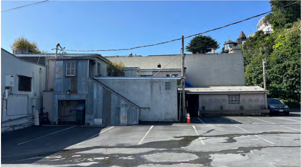
Figure 28: 605 & 607 Bridgeway, north elevations and exterior stair, "Auto" shed on right, looking south from parking lot (Turnbull May 2024)
