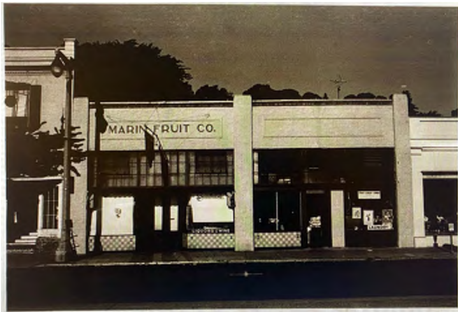
Figure 41: c.1988 around the termination of the Lee laundry, bulkhead tile is still visible on both 605 & 607 Bridgeway (City of Sausalito, digitized building records)
