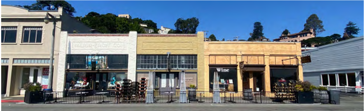
Figure 22: 605 & 607 Bridgeway and 611-613 Bridgeway (Turnbull May 2024)
