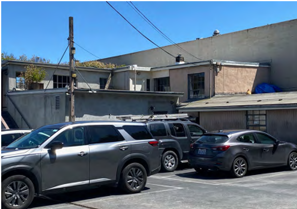
Figure 29: 605 & 607 Bridgeway, north and west elevations, "Auto" shed on right, looking southeast from parking lot (Turnbull May 2024)
