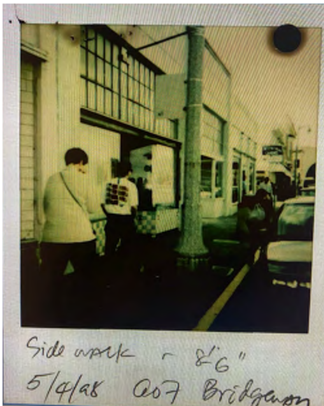
Figures 51: 1998, existing condition at time of proposed storefront alteration (City of Sausalito, digitized building records)
