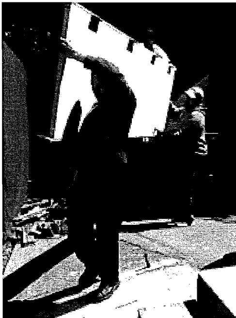
All doors in solid-core untreated poplar, rather than typical doors which are loaded with formaldehyde and layers of glues
