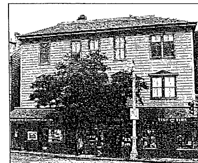
Upper photo: Original condition; note single, double-hung windows at right edge of facade.
