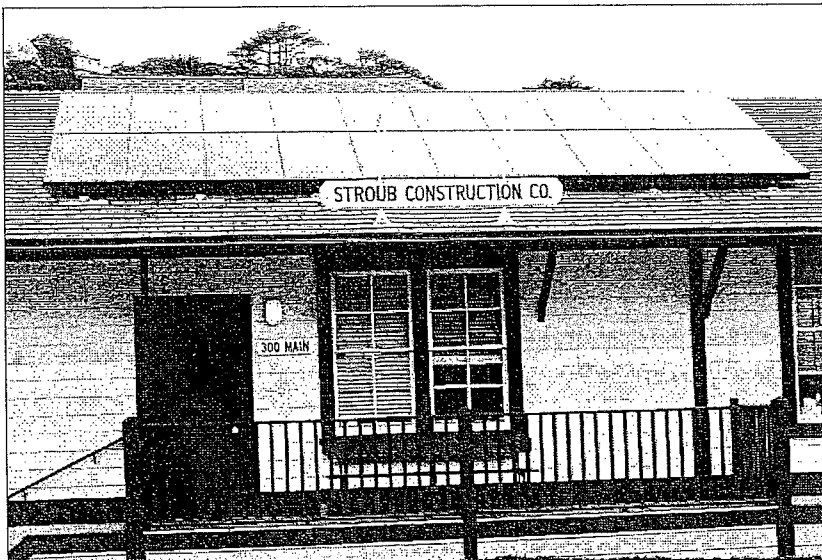
Attach solar collectors to a historic roof in a minimally invasive and reversible manner.
