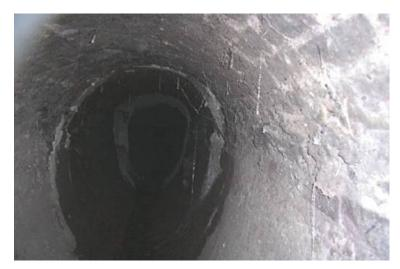
Water can "infitrate" sewer pipes through leaks in pipe joints and connections or through breaks and cracks.
