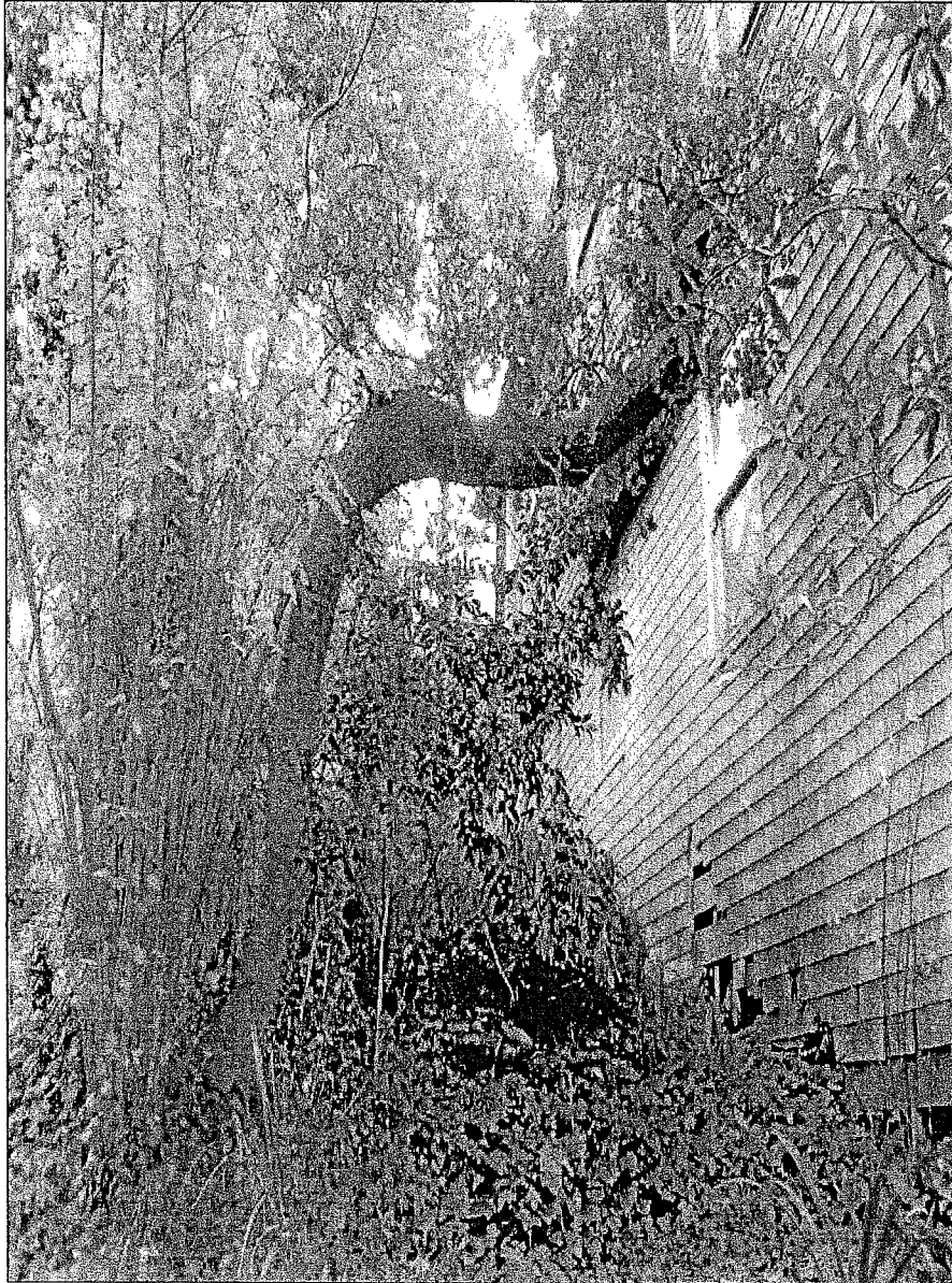
CLO, tree #10, poor structure growth conflict with existing home can not be corrected.
